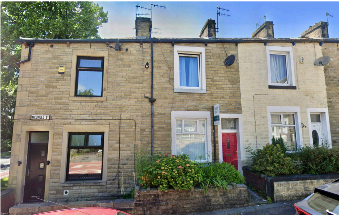
Photograph of front elevation taken from Melville Street.
