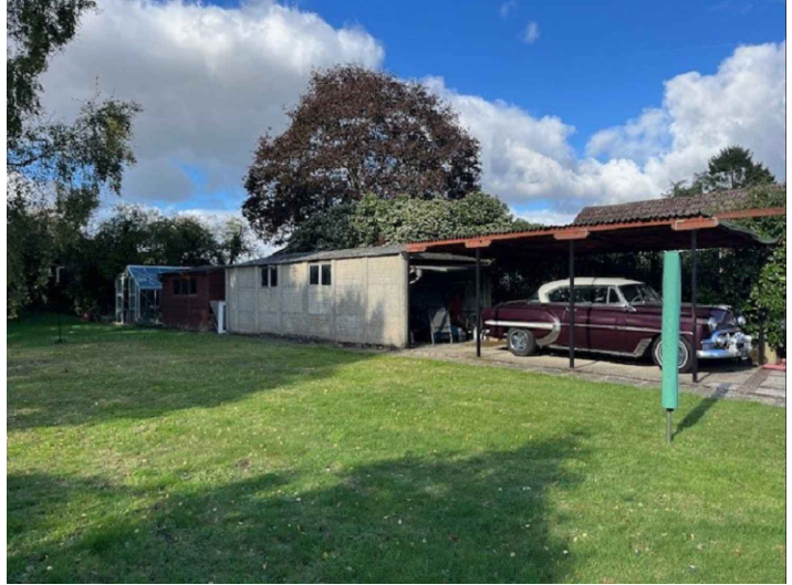
PHOTOGRAPH SHOWING THE EXISTING GARAGE/CARPORT & OUTER BUILDINGS
