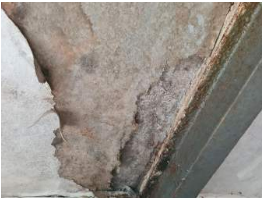
Photograph 10: Garage roof structure of wood ply with felted top surface above.
