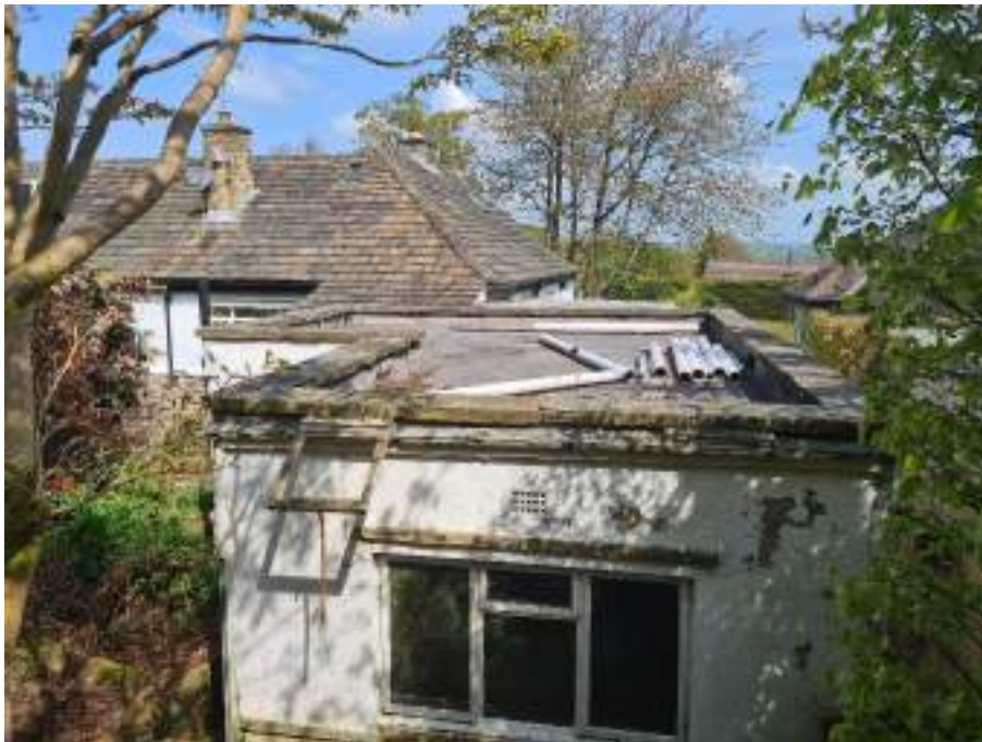
Photograph 11: Garage roof structure of wood ply with felted top surface above.
