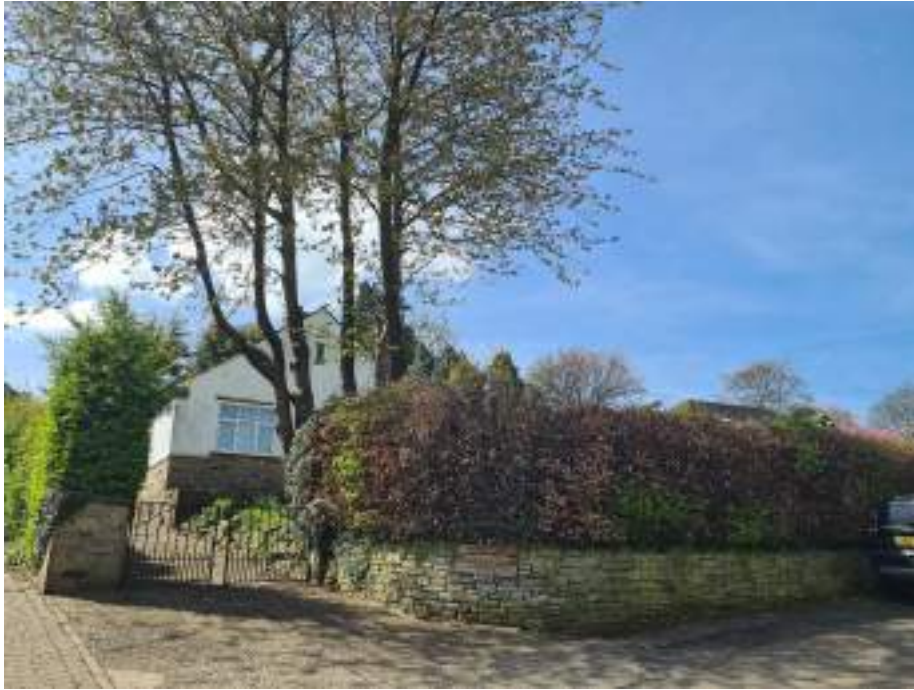
Photograph 1: A view of the property as taken from the roadway of St. Giles Garth.
