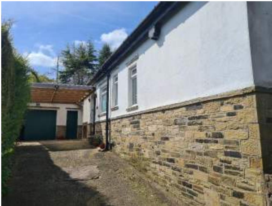
Photograph 7: Side elevation of the property noting construction of local Yorkshire sandstone.
