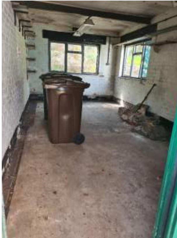
Photograph 9: An internal view of the garage. Noted clean concrete flooring and no storage of potentially hazardous materials.
