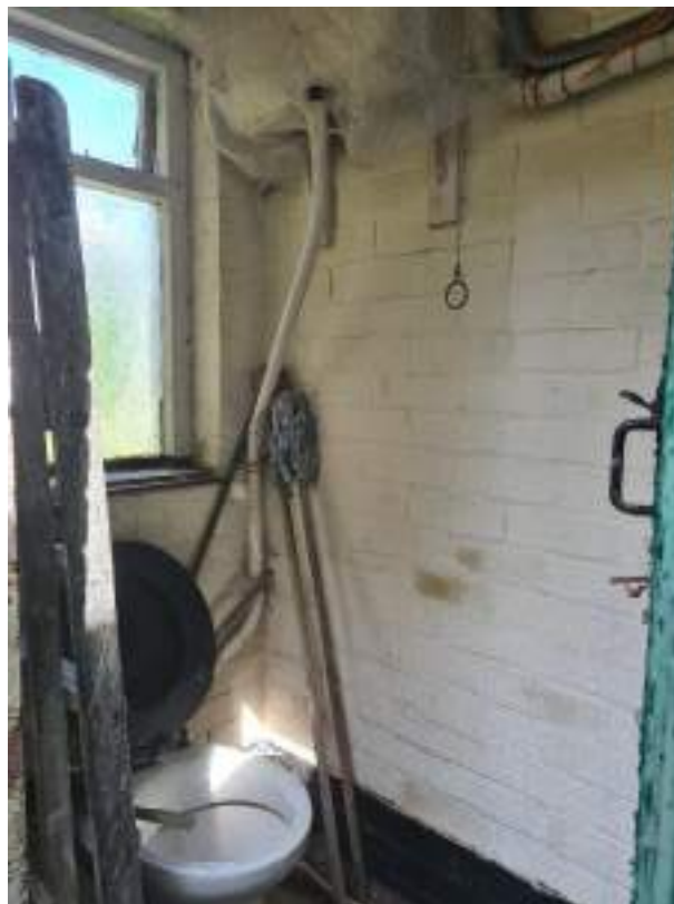
Photograph 12: Small disused toilet to the rear of the garage.
