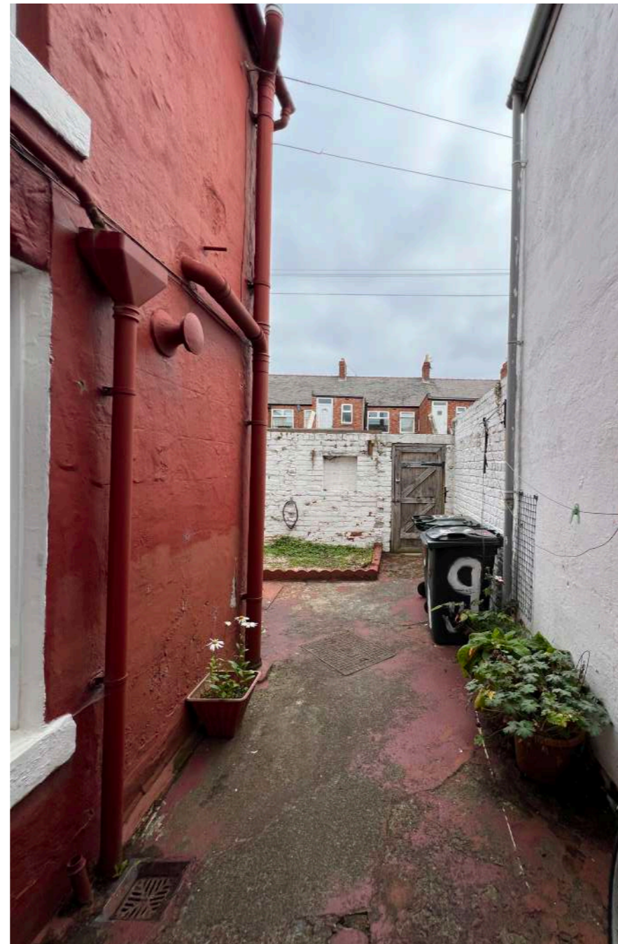
4 / View from kitchen door
