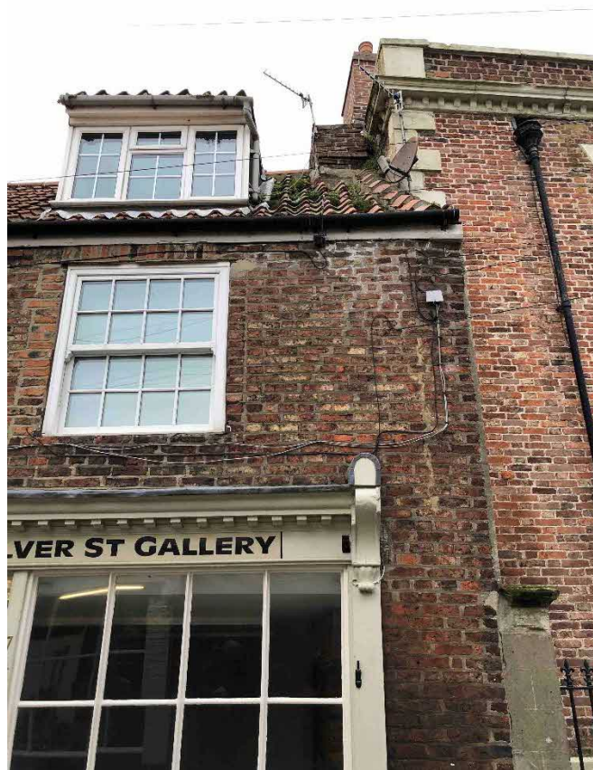
Photo 4 North end of roof, brick stub chimney
