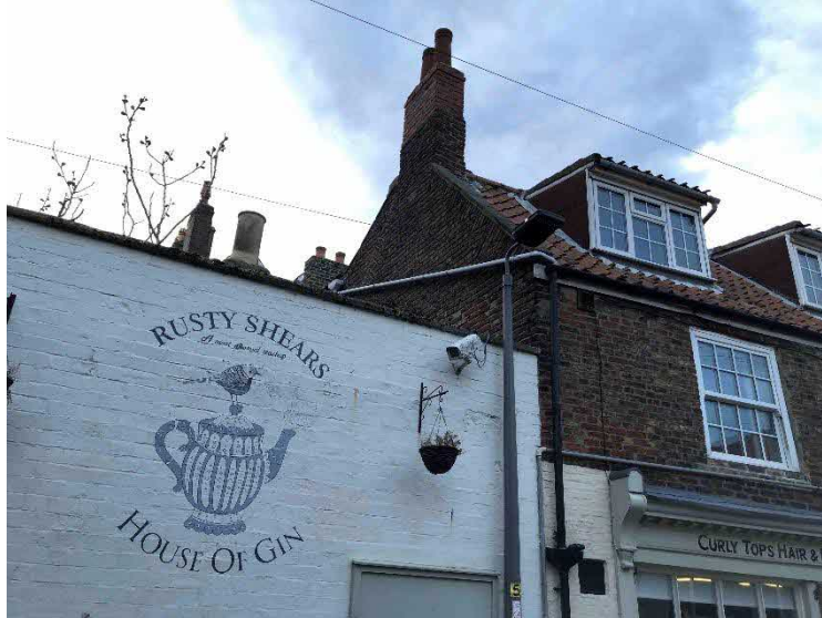
Photo 3 South gable, dormer detail and chimney
