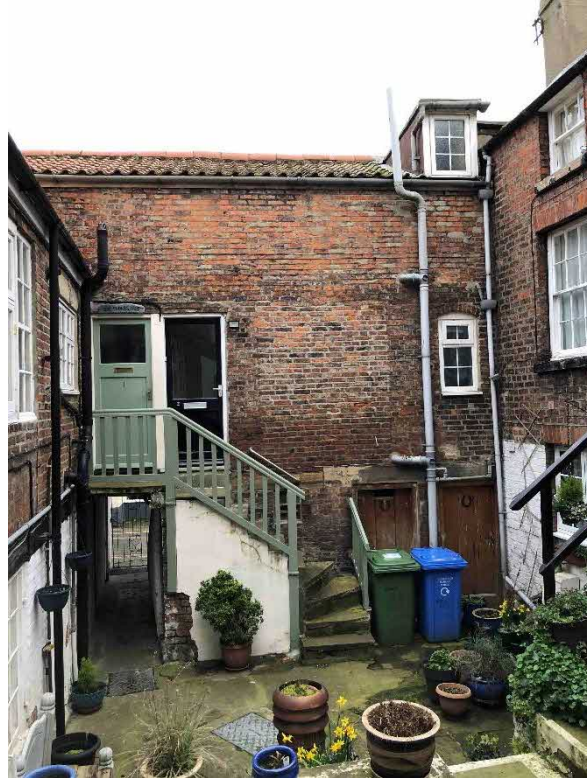
Photo 5 Rear elevation from Elders Yard
