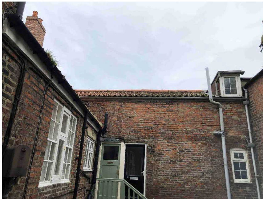
Photo 6 Rear elevation detail of dormer and raised brickwork
