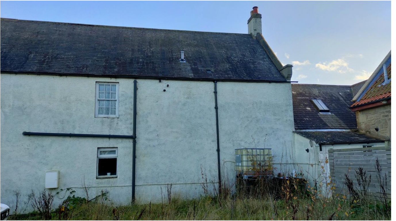
Site Of ASHP (at existing oil tank)
