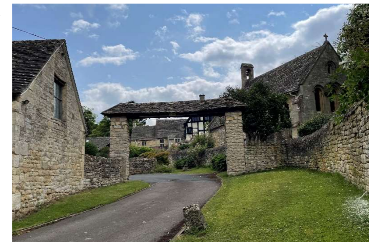
Fig 19 (top) The church viewed from the former farm yard looking east. Fig 20 (middle) The church, 1951, Fig 21 (above) View from the private drive into the picturesque group.
