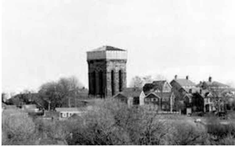
the tower with watertank [before demolition]
