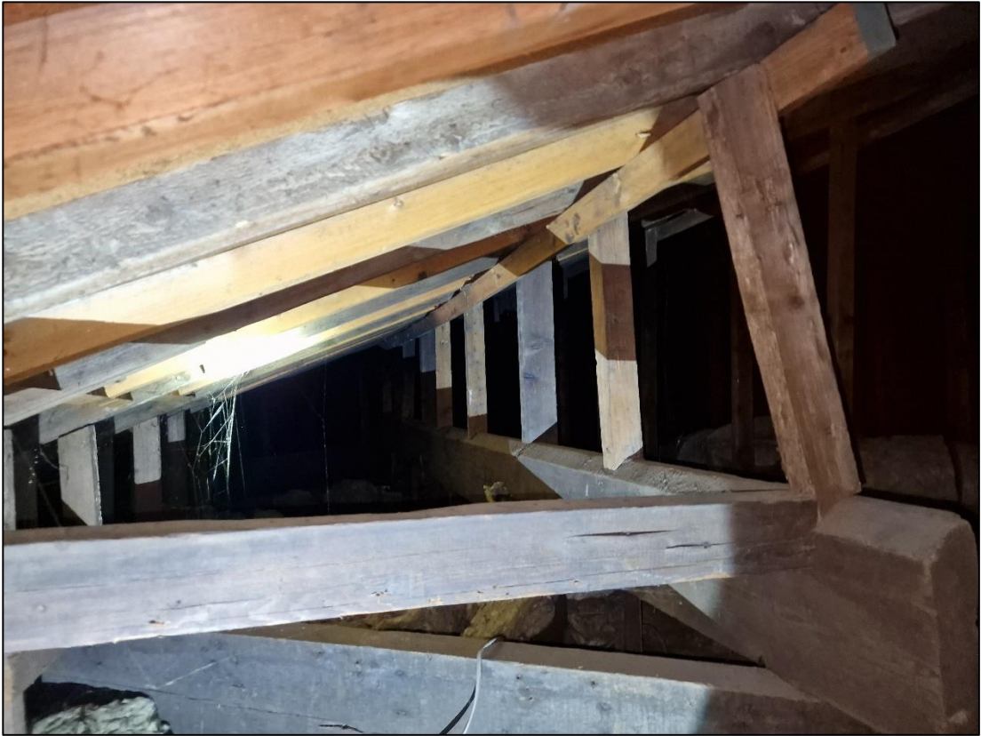
Plate 1 – The general character of the internal voids of B1
