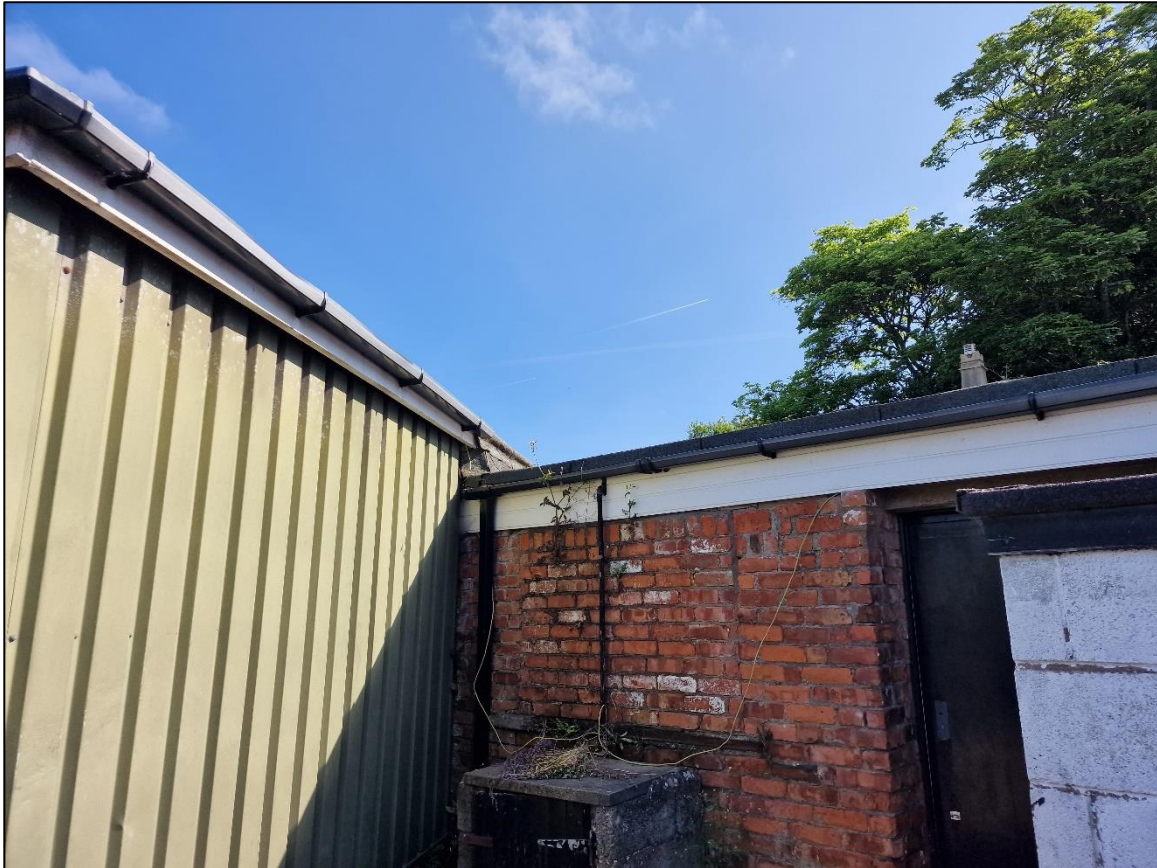
Plate 5 – General character of the gap behind the barge boards at the wall plate level; note the floodlight
