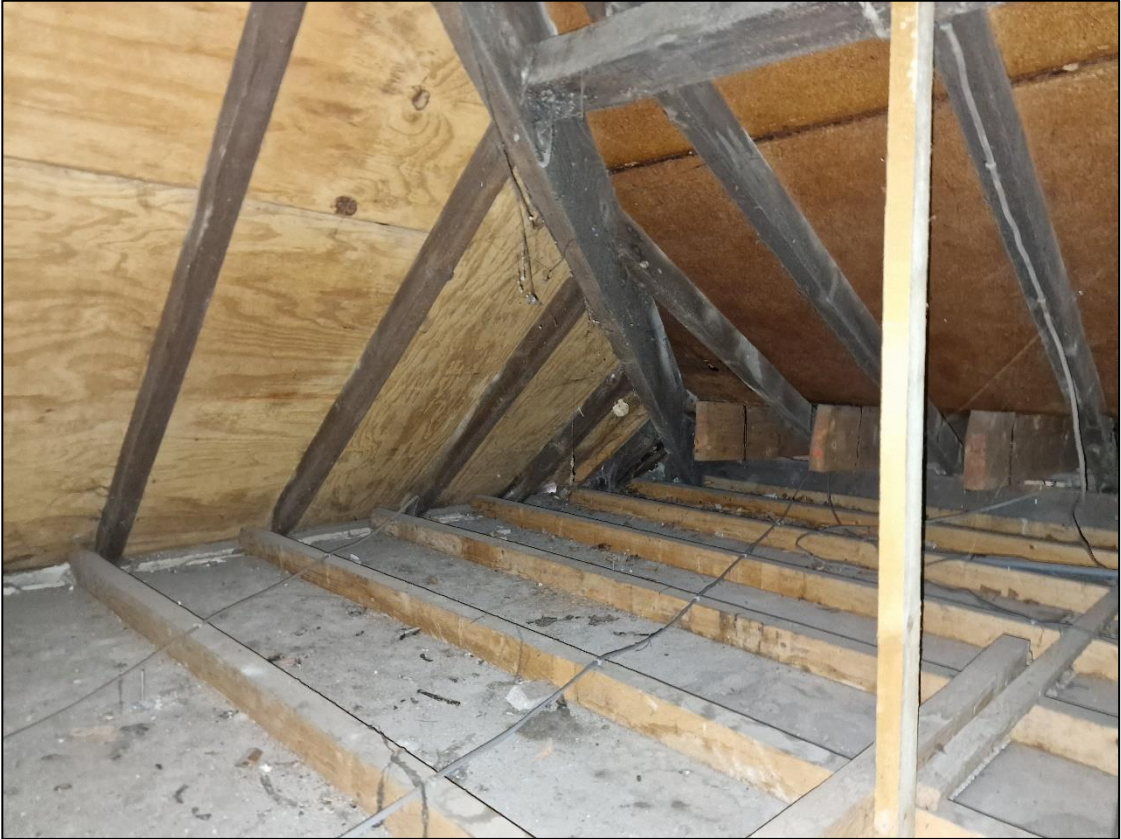
Plate 2 – Additional aspect showing the internal void of B1
