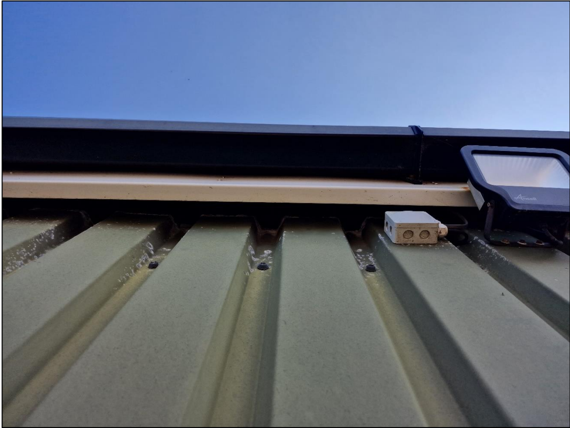
Plate 5 – General character of the gap behind the barge boards at the wall plate level; note the floodlight
