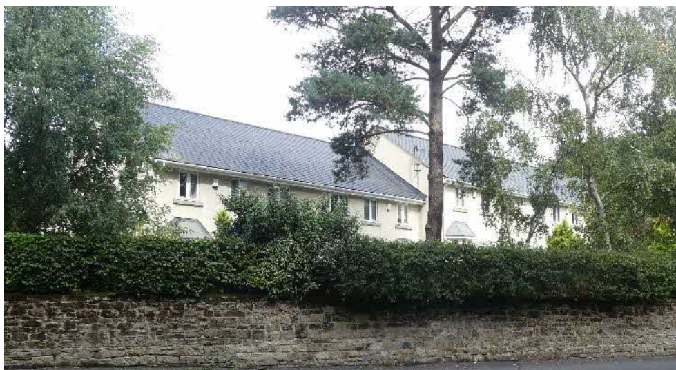
Figure 2.26: The recent residential development on the northern side of Damfield Lane
