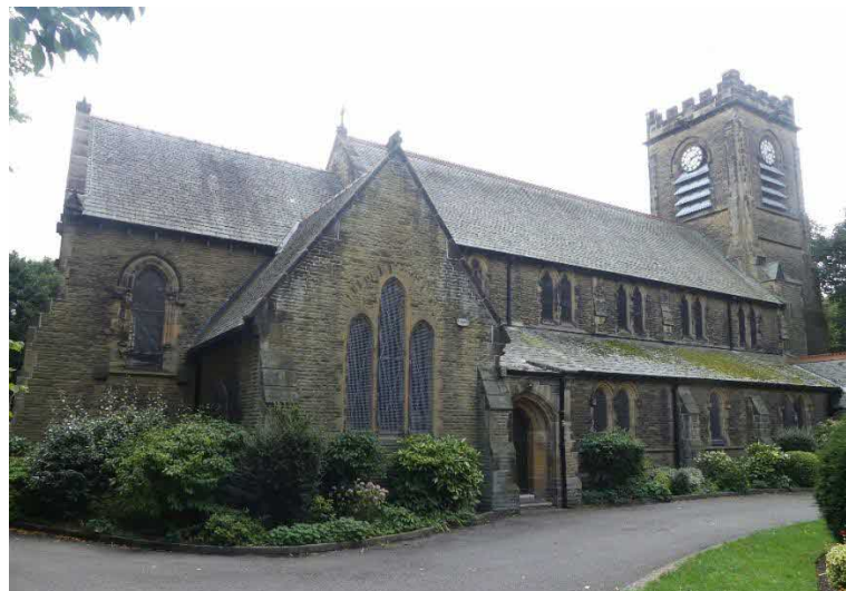
Figure 2.1: The northern elevation of St. Andrews Church
