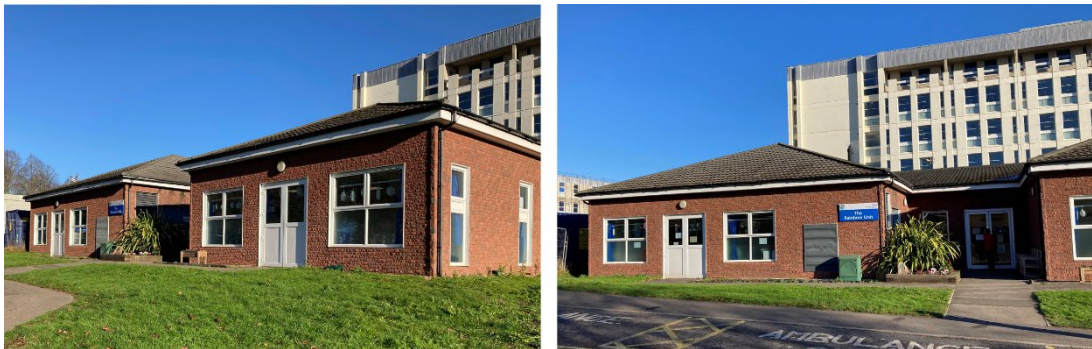
Figure 2 – Views to the front of the building
