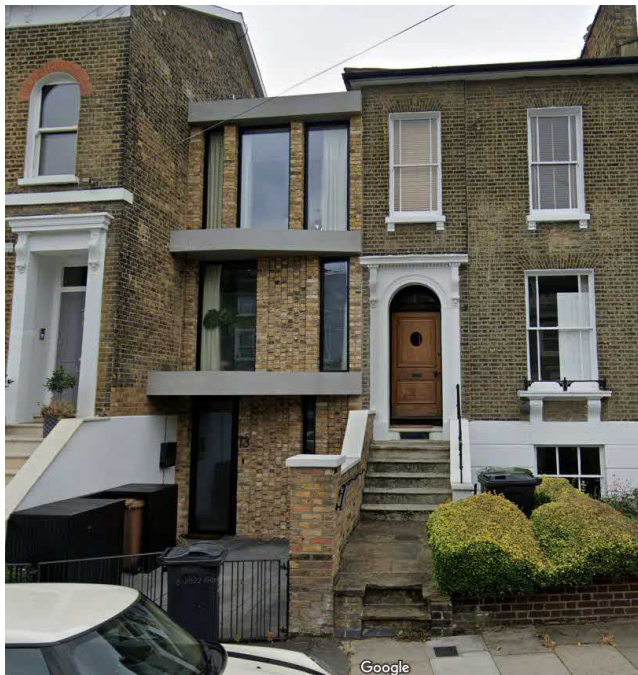
St Donatts Road – This example shows the flat roof was approved by stepping it from the main roof. However, there is no step back from the principal elevation.
