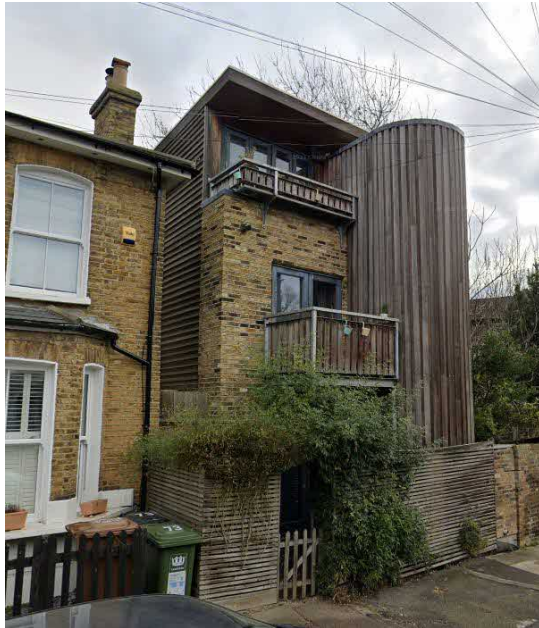
St Donatts Road – example of Timber cladding and a flat roof approved in the area. Along with leaving a alley way between the two properties
