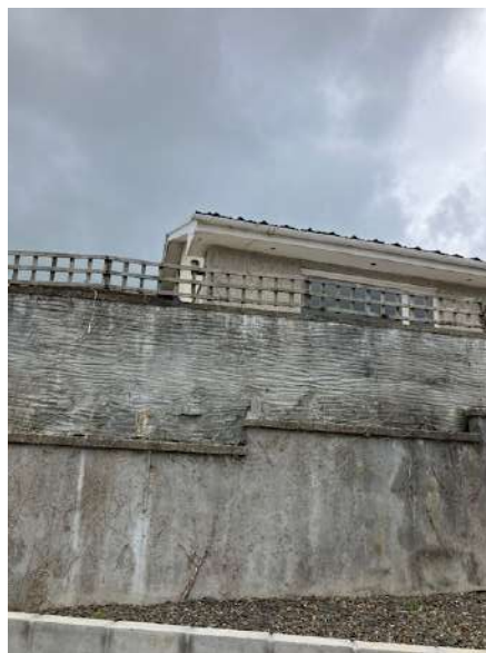
Retaining wall of adjacent property
