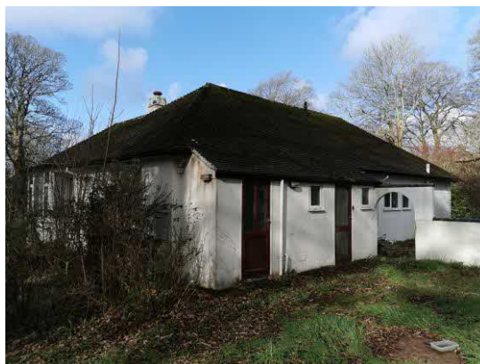
Photo 3. Showing the building from the south east
