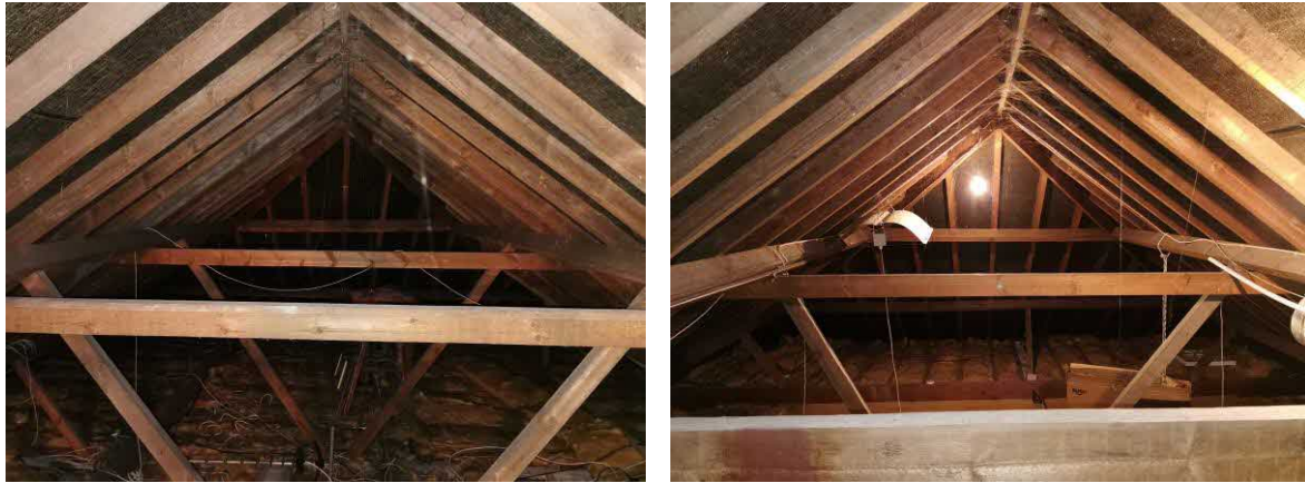
Photos 4 and 5. Showing the roof void over the building
