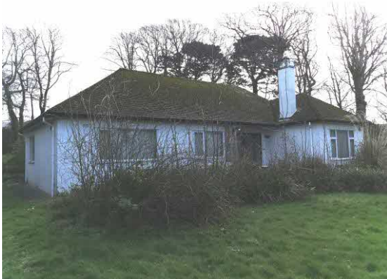
Photo 1. Showing the building from the north west
