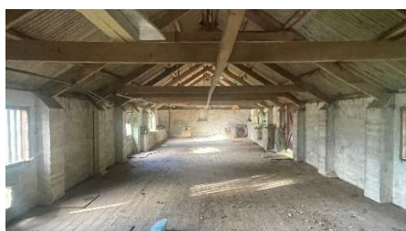
First floor view of barn interior
