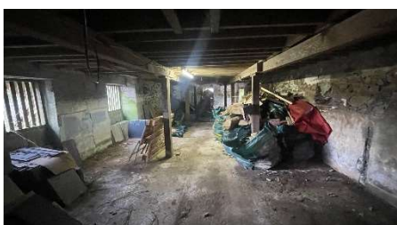
Ground floor view of barn interior
