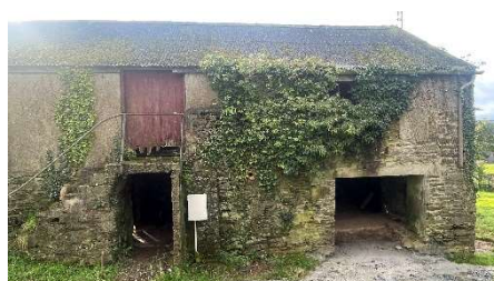
West end of barn facing drive
