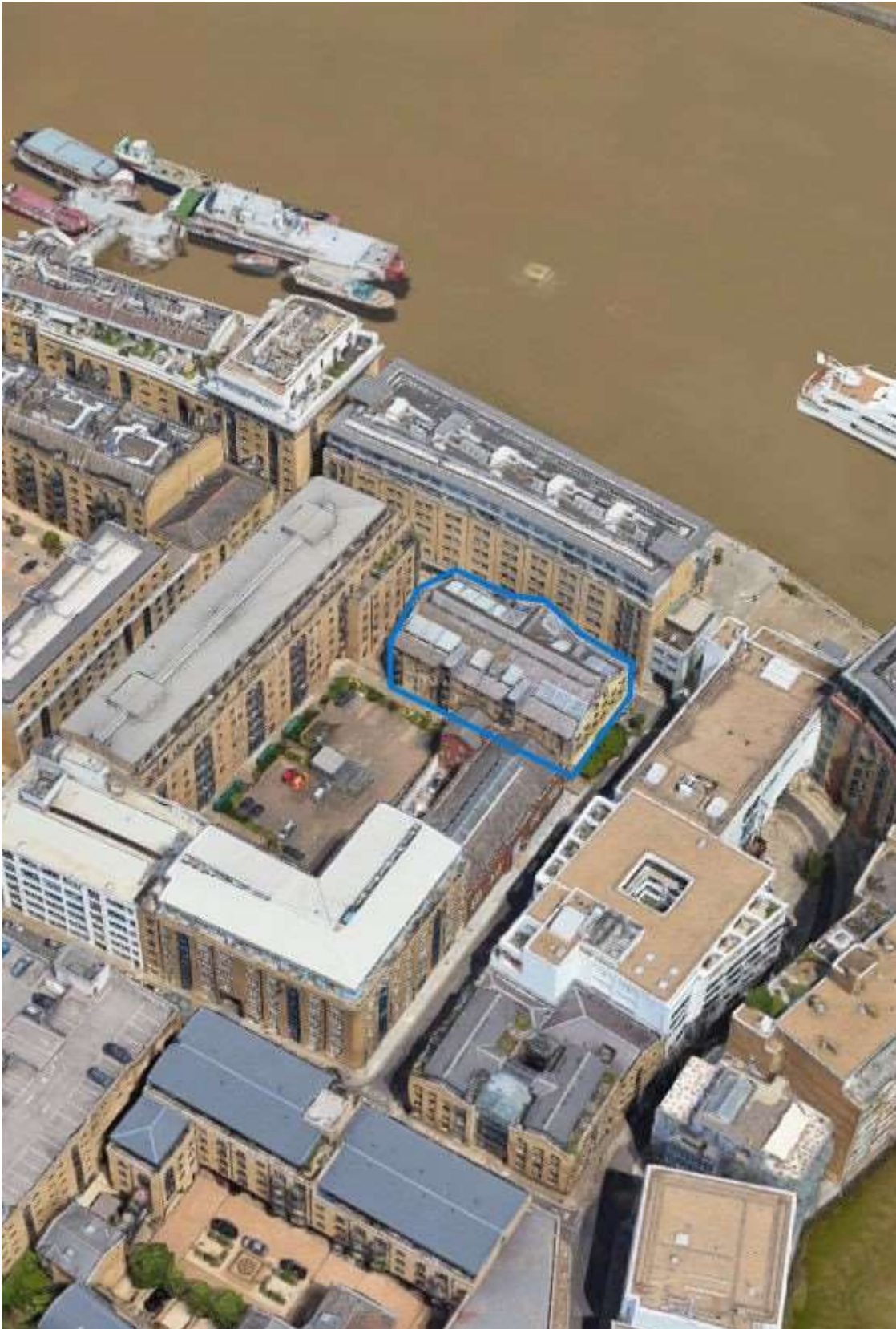
Aerial view with Wheat Wharf building outlined
