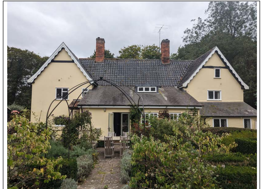
The rear of Park Gates
