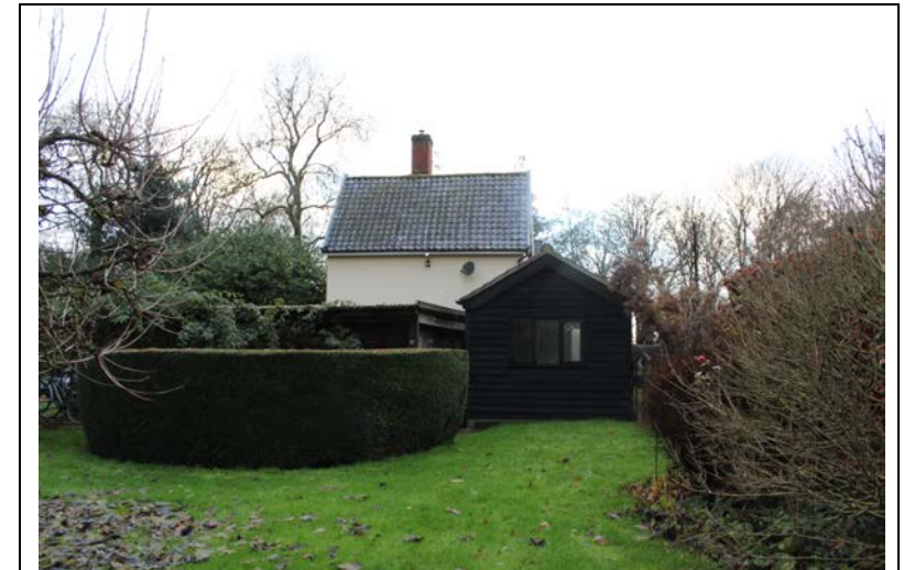
Matching materials will be used on the garden studio extension so it appears as a single, long form.
