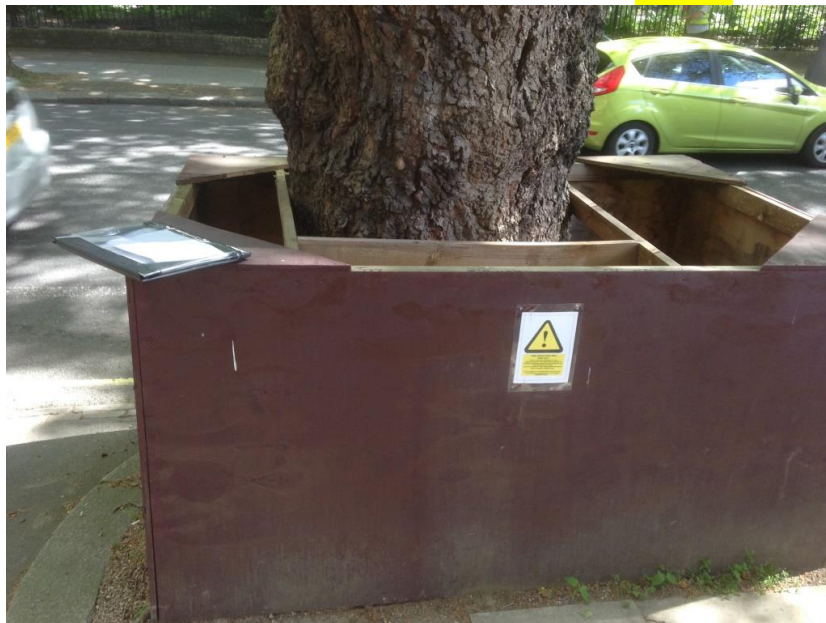
Photo to show example braced heavy-duty ply-board (trunk & tree pit protection) sheeting Tree Protection Box that would be used around T1 and T2
