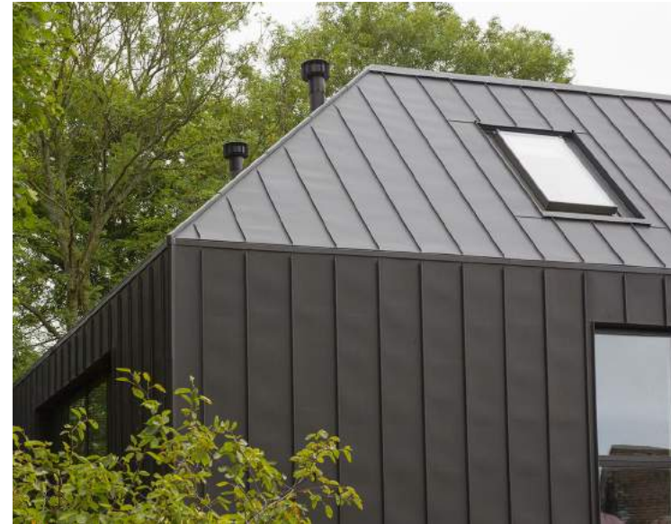
Vertical standing seam cladding
