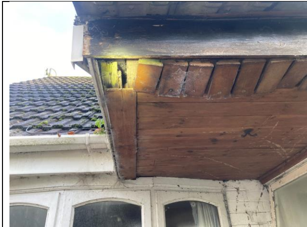
Photo 7 PRF porch soffit
