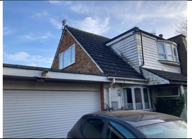
Photo 2 North west gable
