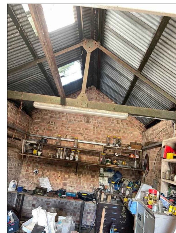
Internal view of metal truss & roofing sheets
