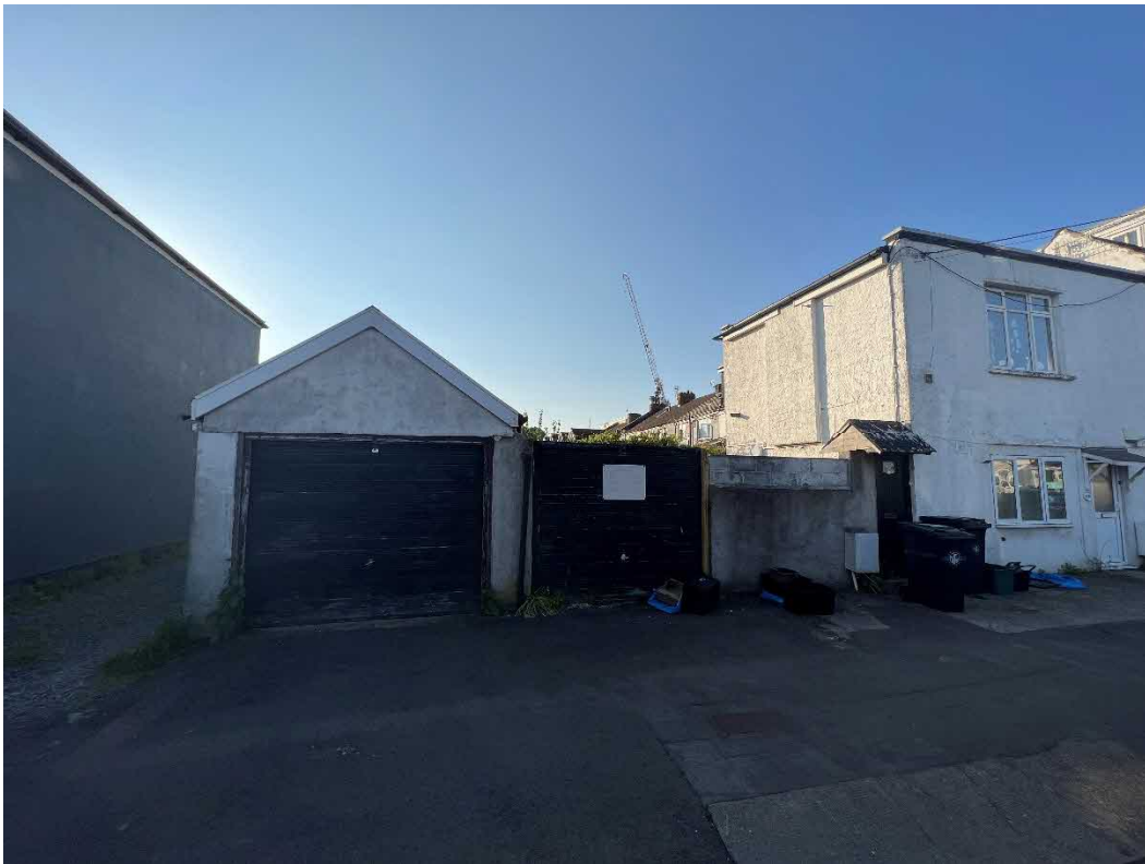
The front elevation – The Garage to the existing building wall.
