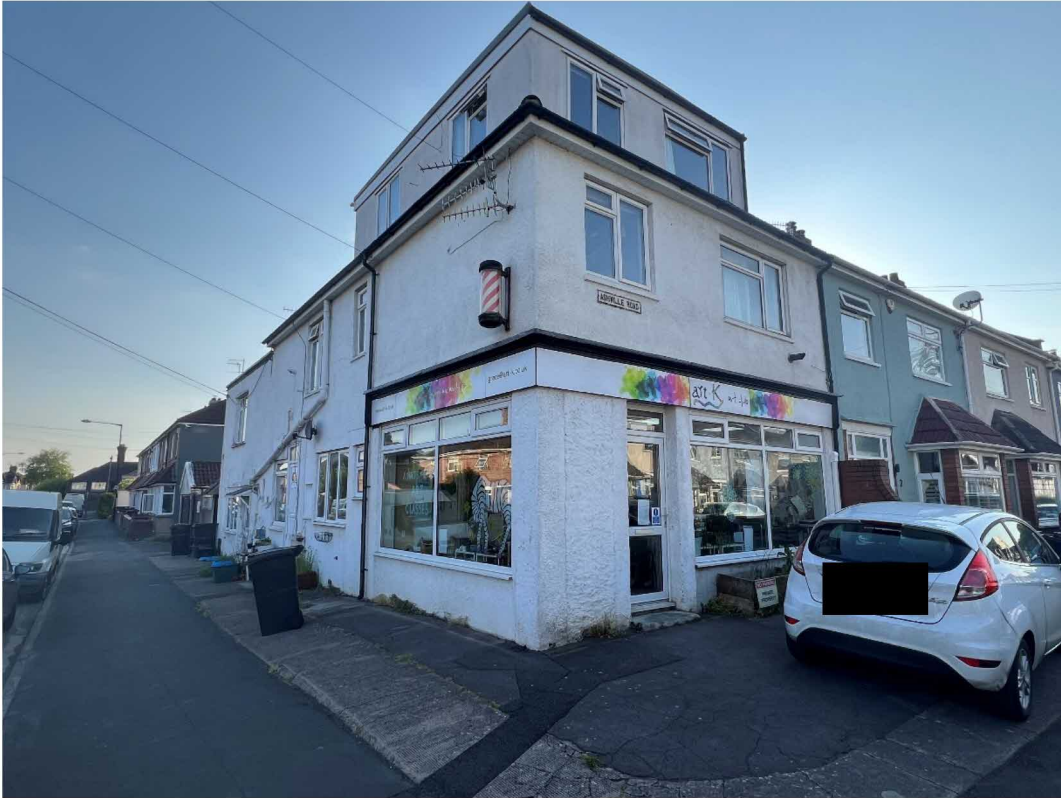
Looking at an angle at the site and the existing building and down the roads
