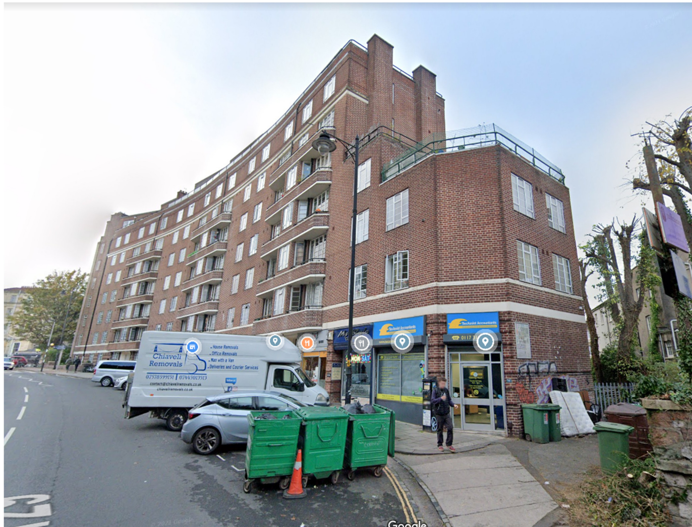
Fig 1- Existing view of Queens Court showing debris and refuse bins
