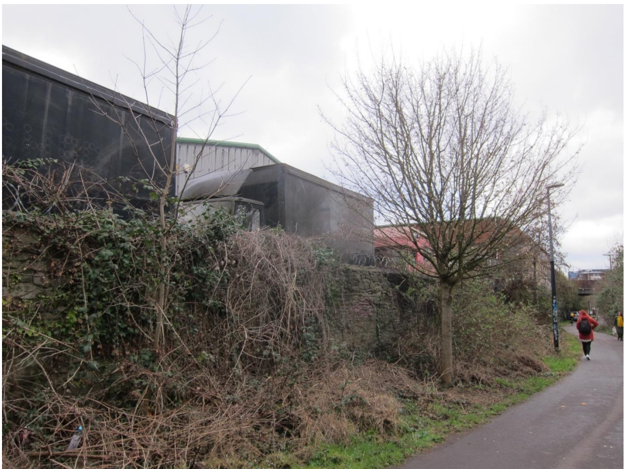
Photograph 1: T8, T9 and G11 from left to right, viewed from the north-east.
