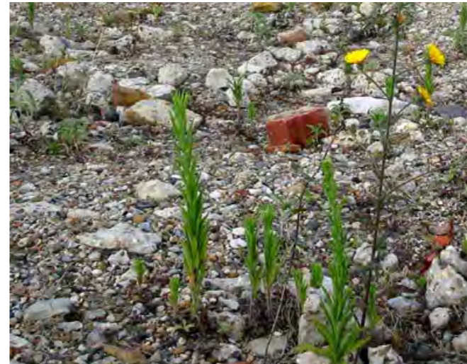
Typical brown roof
