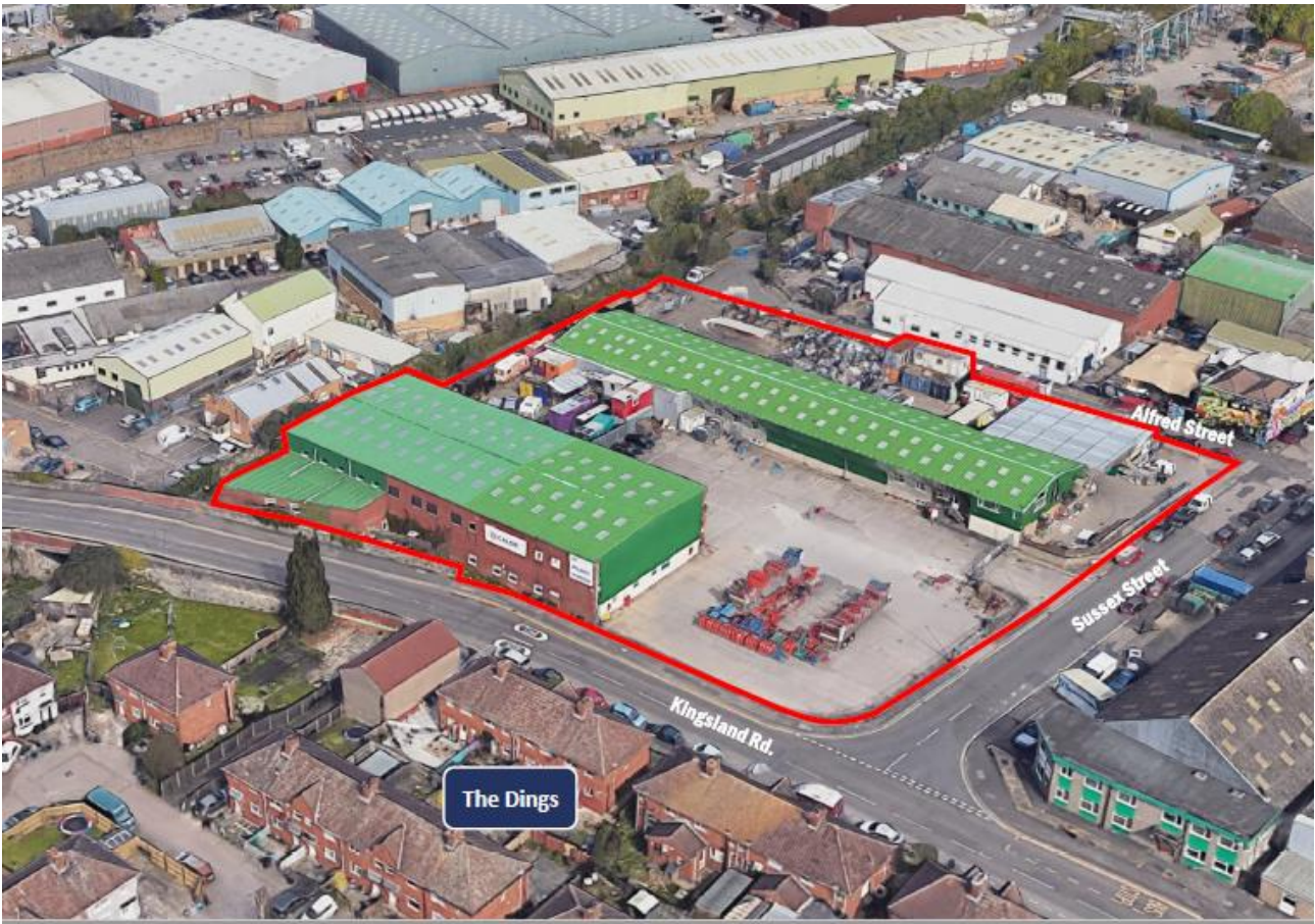
Figure 1 – View of the existing site and the surrounding area
