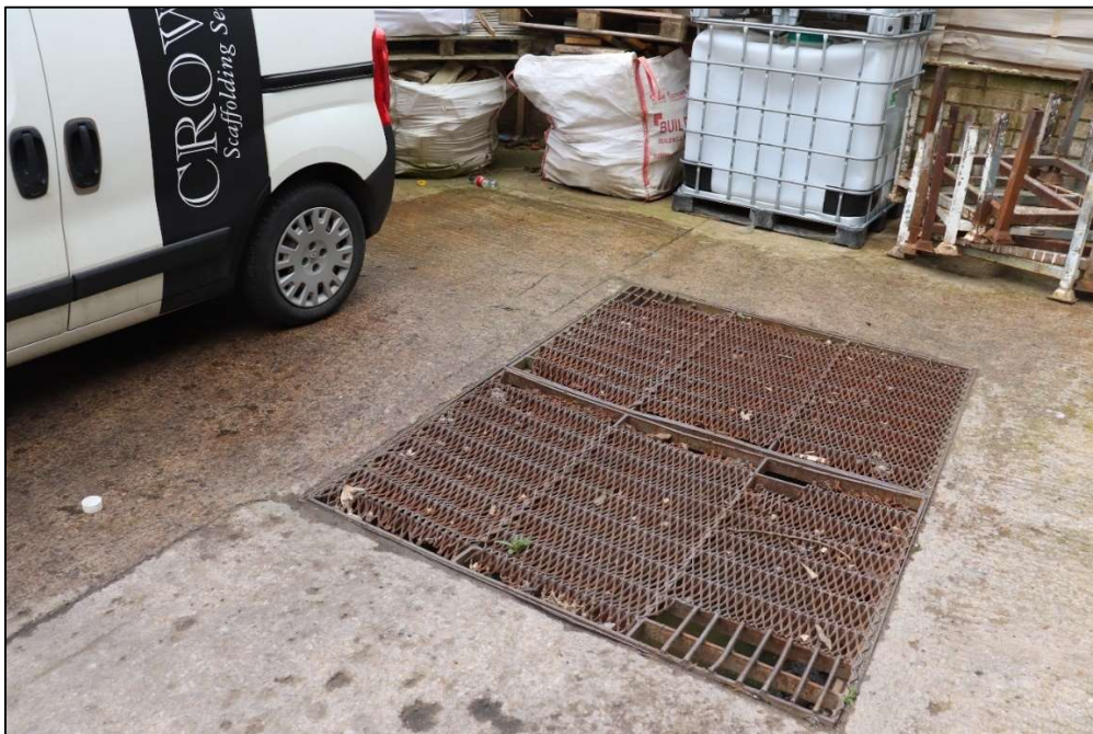
Inspection pit in the yard of Crown Scaffolding, March 2023
