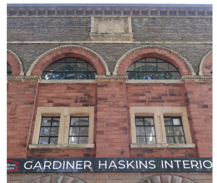
Polychromatic stonework with a base and top of grey Pennant stone with red sandstone and buff limestone, Gardiner's Warehouse (Gardiner Haskins), 1884
