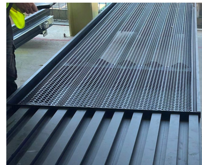
Perforated corrugated metal vent panel above a ribbed fixed panel, from a different AHMM project (not intended for colour reference, to be conditioned).
