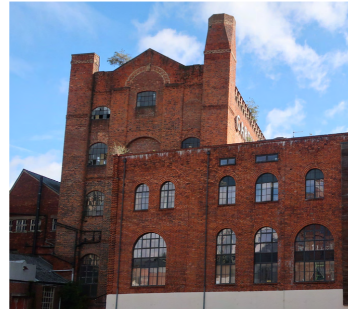
Orange/red brick at Gardiner's Warehouse (Soapworks), Straight Street (1841-1882)
