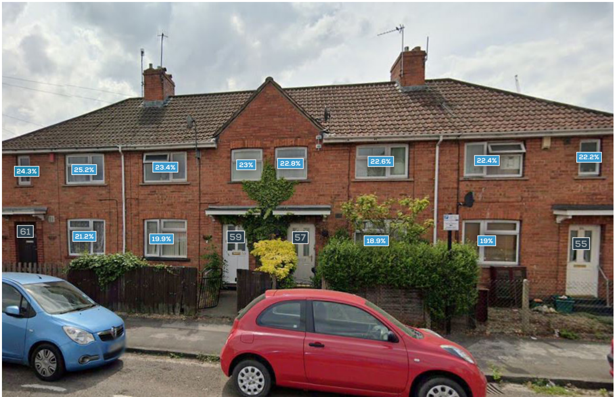
Figure 05: Window Map highlighting the proposed VSC values to those windows which do not meet the BRE's recommendations for VSC
