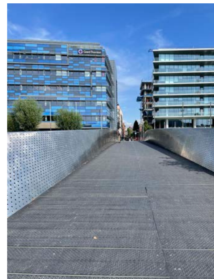
Figure 5.10: Meads Reach Bridge.
