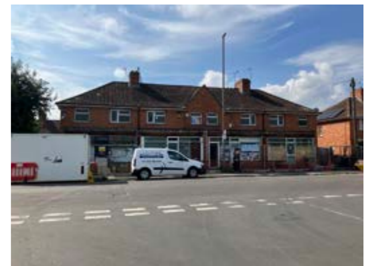
Figure 5.2: 63-69 Kingsland Road, an example of the fine-grain, semi-detached housing found within the Dings.
