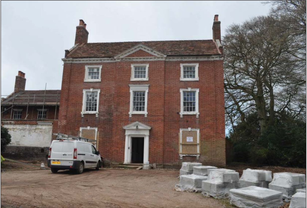
Plate 1 - Grade II listed Ismere Hall front elevation
