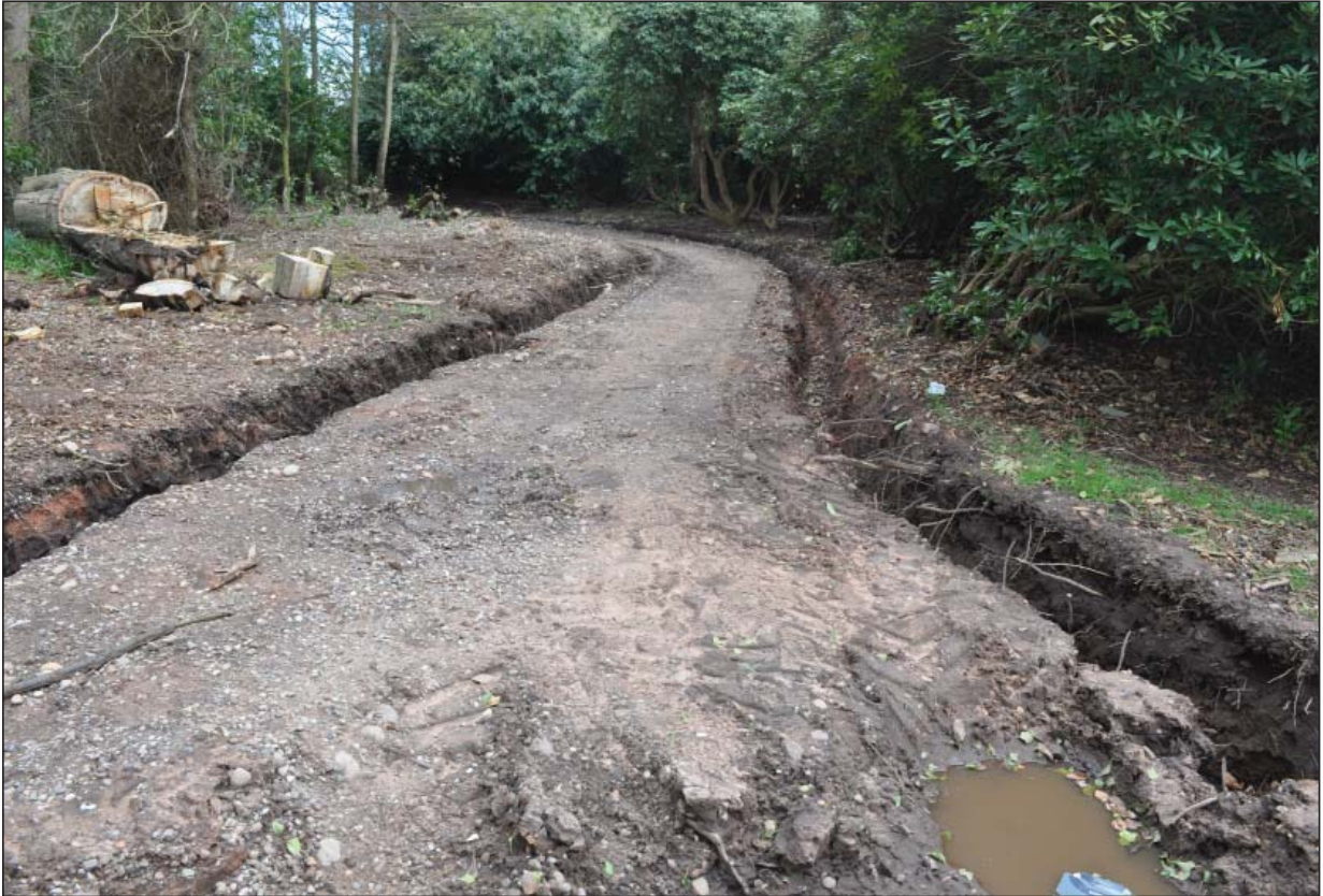
Plate 7 - Service trenches in eastern driveway
