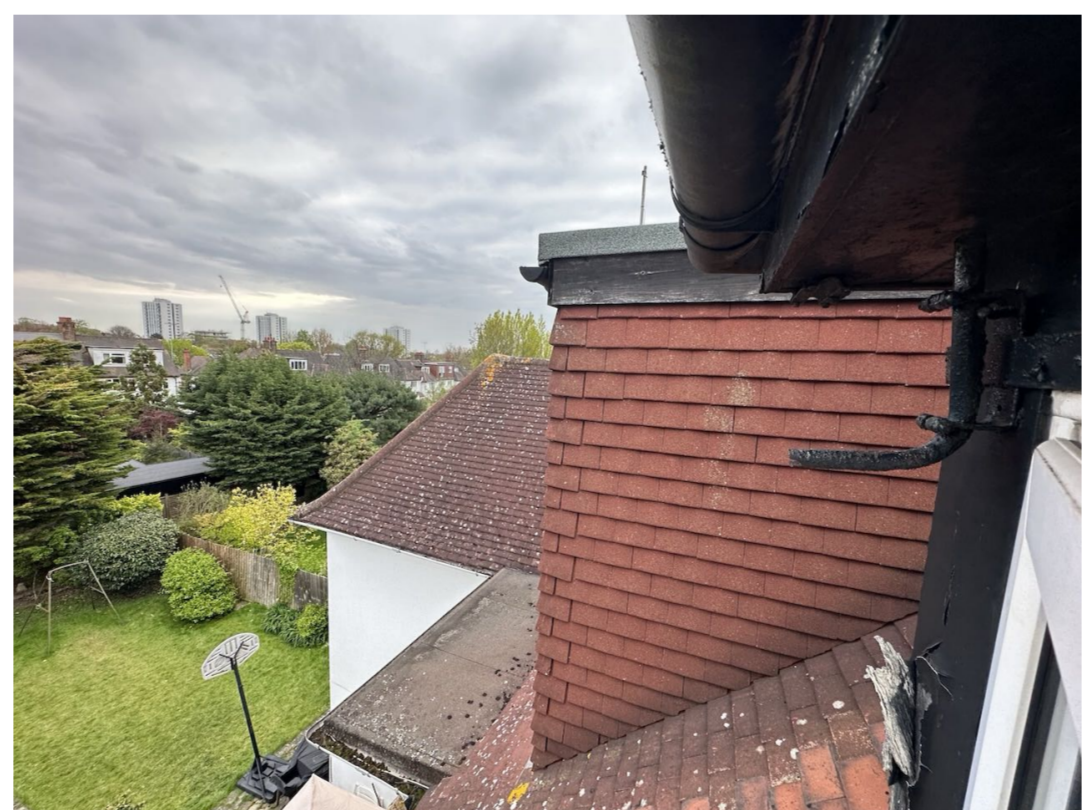
View from N°13 dormer looking towards N°15 dormer
