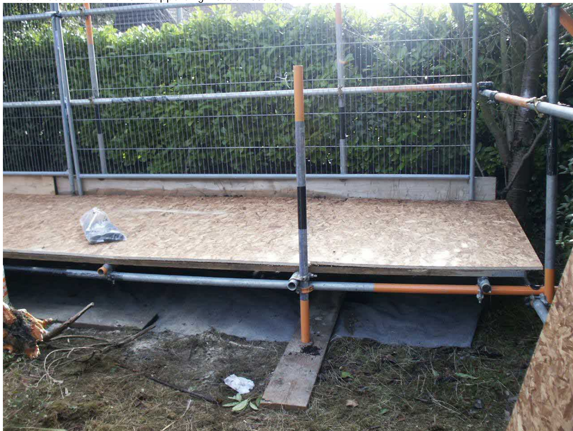
Photo 2 Scaffold framework supporting wooden boards
