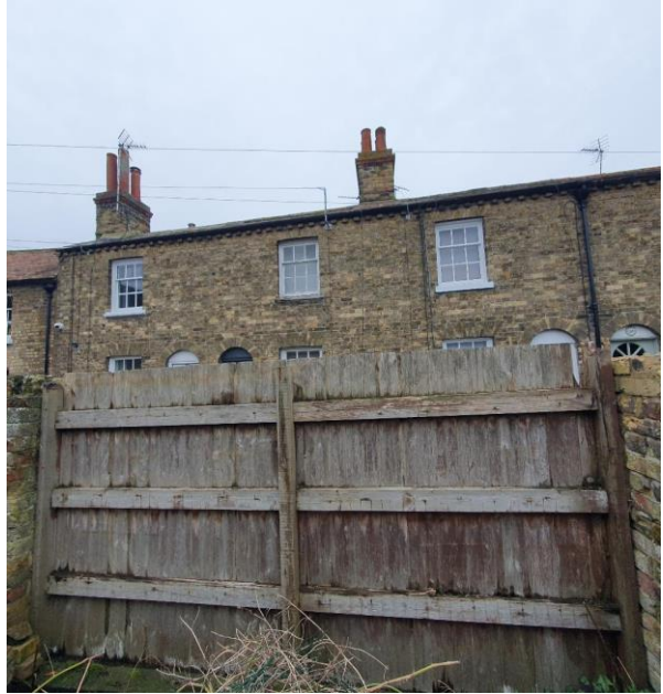
Fig. 6 Vehicle Access Gate
