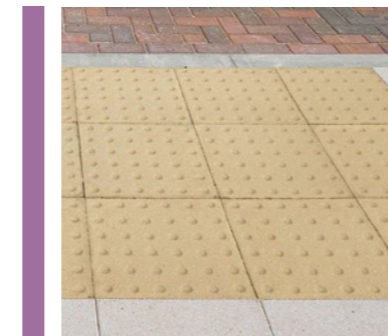
Proposed tactile paving Marshalls Tactile Blister paving Colour: Charcoal Size: 400 x 400mm
