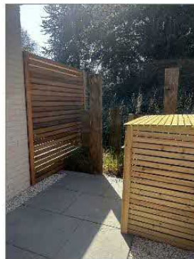
Photograph 1 Installed 2.0m slatted fence to side of terrace.
