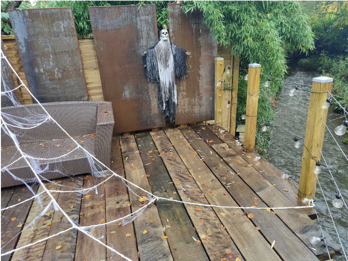
Photos 1 and 2 – The new decking
