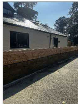
Photograph 2 Installed 0.5m fencing on existing boundary wall.
