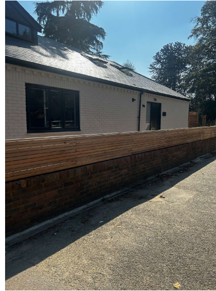
Photograph of Fencing to Boundary Wall at Front Elevation
