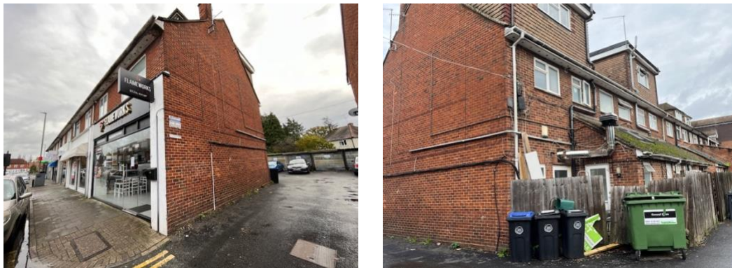
Figure 4 - 27 Frimley High St front and rear facades
