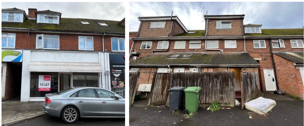
Figure 2 - 25 Frimley High St front and rear facades
