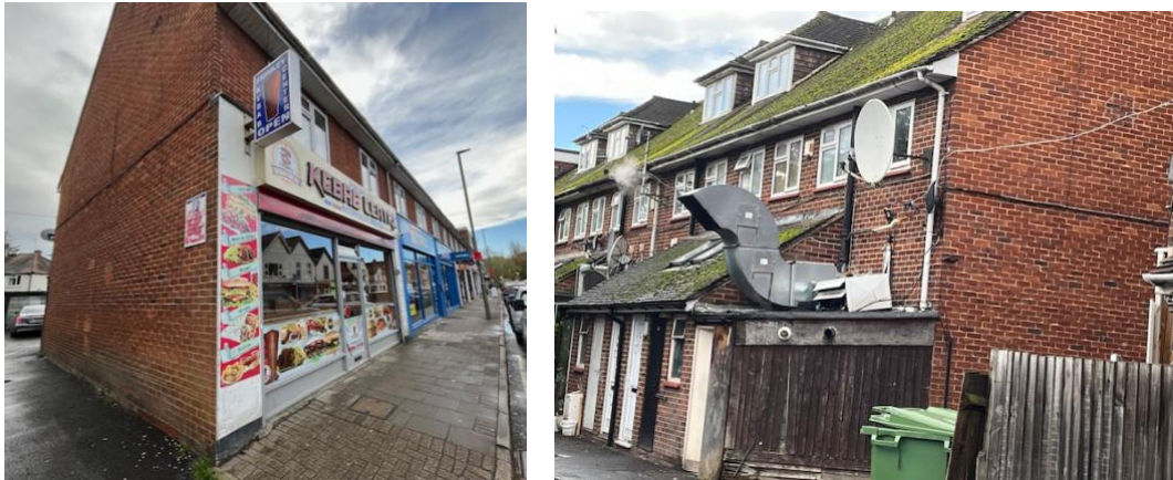
Figure 3 - 29 Frimley High St front and rear facades
