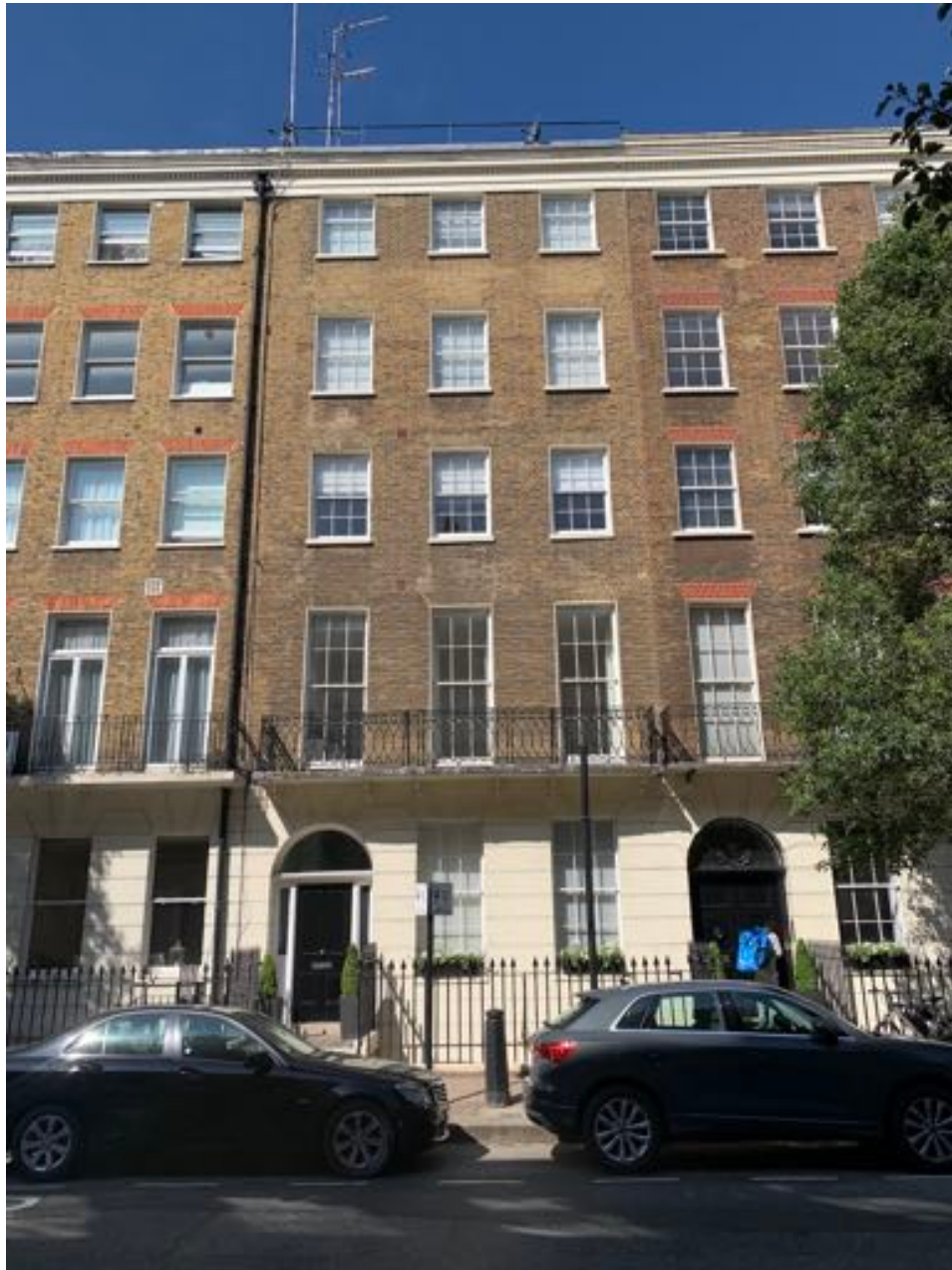
Photo A : front elevation of 57 Great Cumberland Place.
