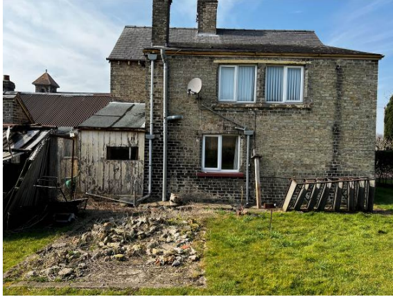
Rear of house showing timber Kitchen construction
