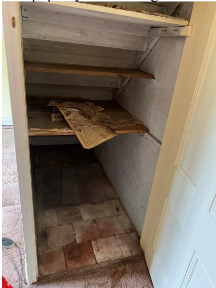
Damp quarry tile flooring
