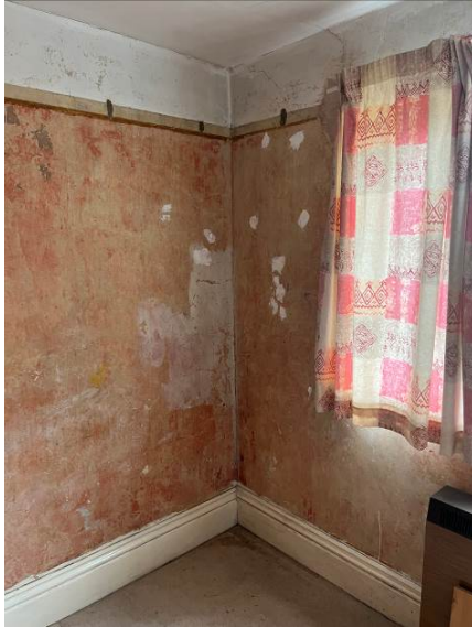
Damp external wall Bed 1
