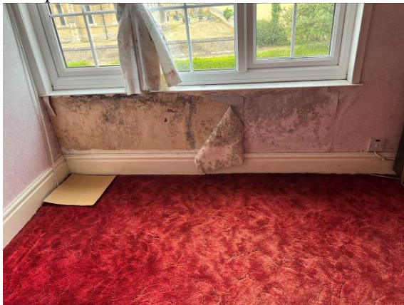
Damp external wall Bed 1
