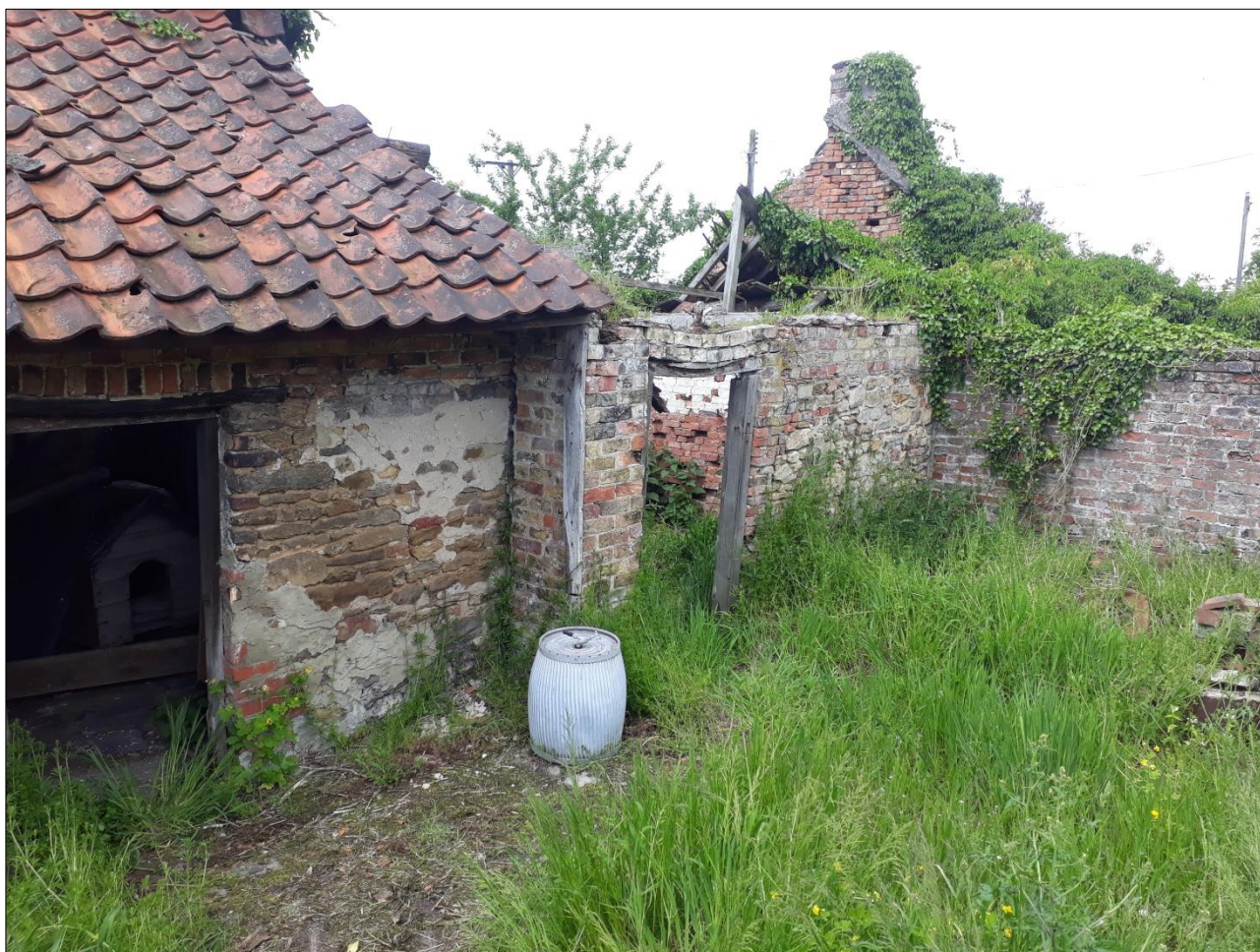
Outbuildings looking northwest. On the left is an earlier stone-built agricultural building, later extended in brick (centre and right). Ivy covered chimney to right served a small metal-working hearth and copper for heating water, neither of which are intact
