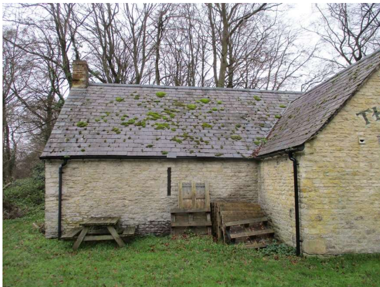
Photograph 2 – eastern end of north facing front elevation, fully tiled and hips close bedded
