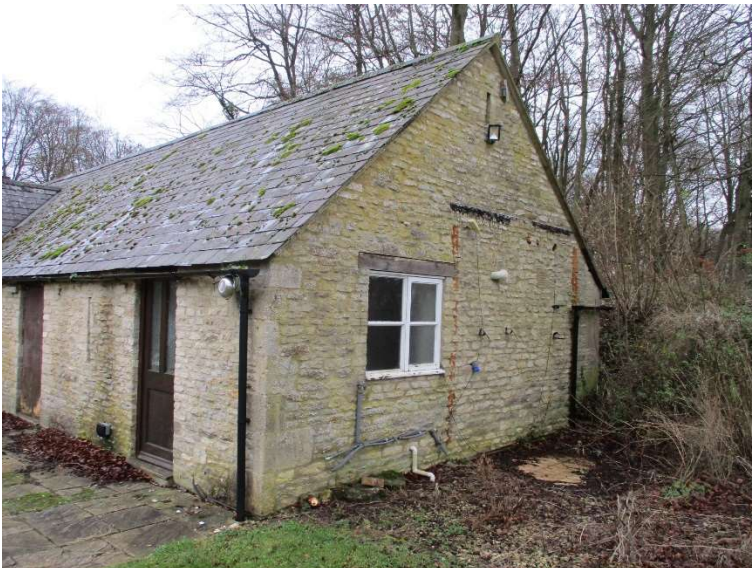
Photograph 6 – western gable end with eaves details all closed.
