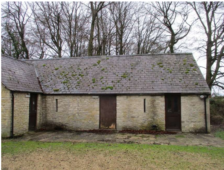
Photograph 4 – western end of north facing elevation with closed eaves, ridge and sealed openings
