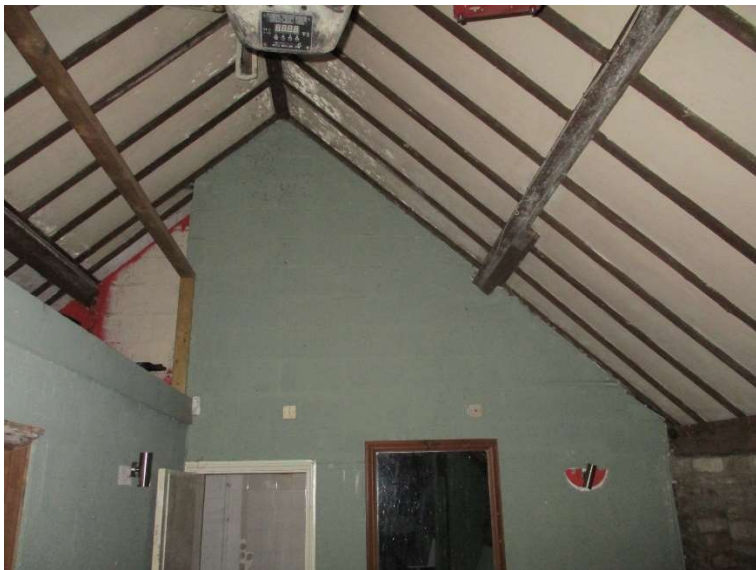
Photograph 8 - inside looking west, note ceilings closed, no roof void and no indication of bird or bat activity.
