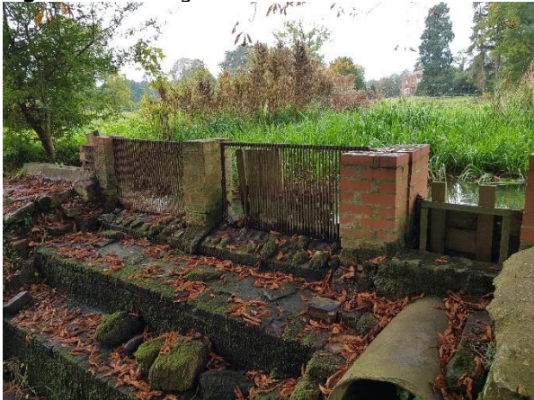
Figure 20 East side of the weir from the north bank showing various materials used for construction.
