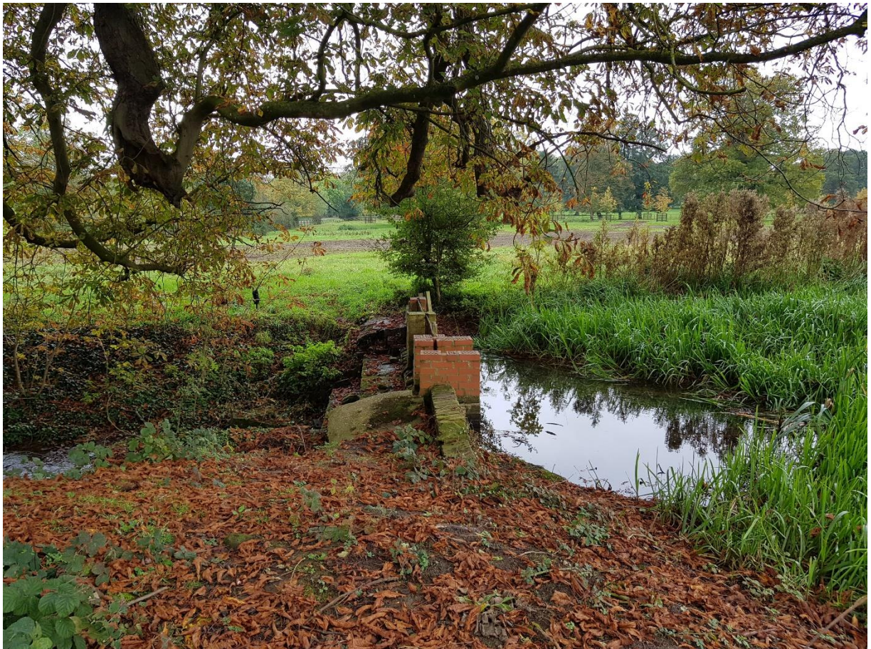
Figure 17 Looking south along the line of the weir.
