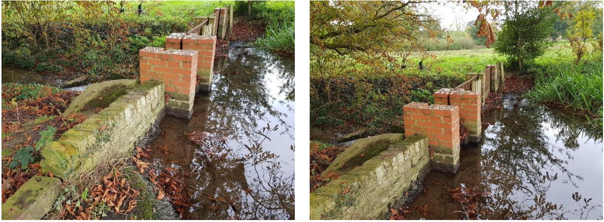
Figure 21 Looking southeast across the back (west side) of the weir.
