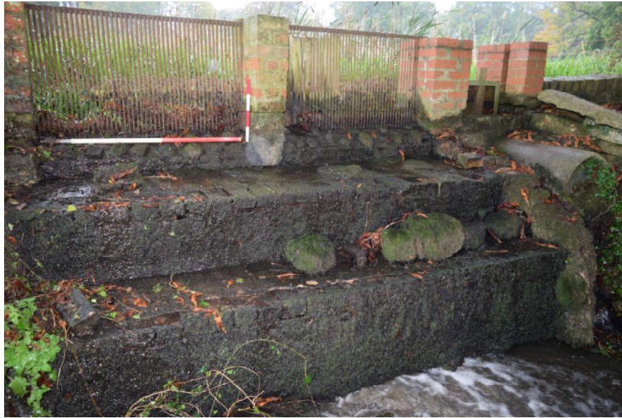
Plate 2: View of the weir, looking west. Scales are 1m and 0.4m
