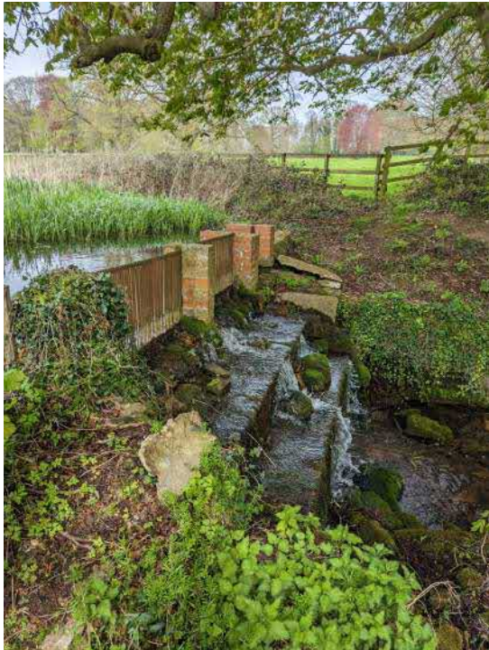
Fig 10. Downstream view of the weir from south bank
