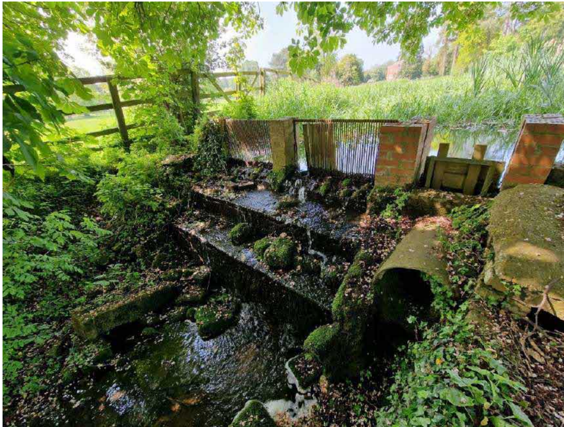
Fig 11. Downstream view of the weir from north bank
