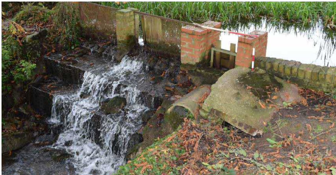
Fig 12. Existing weir viewed from downstream when operating normally
