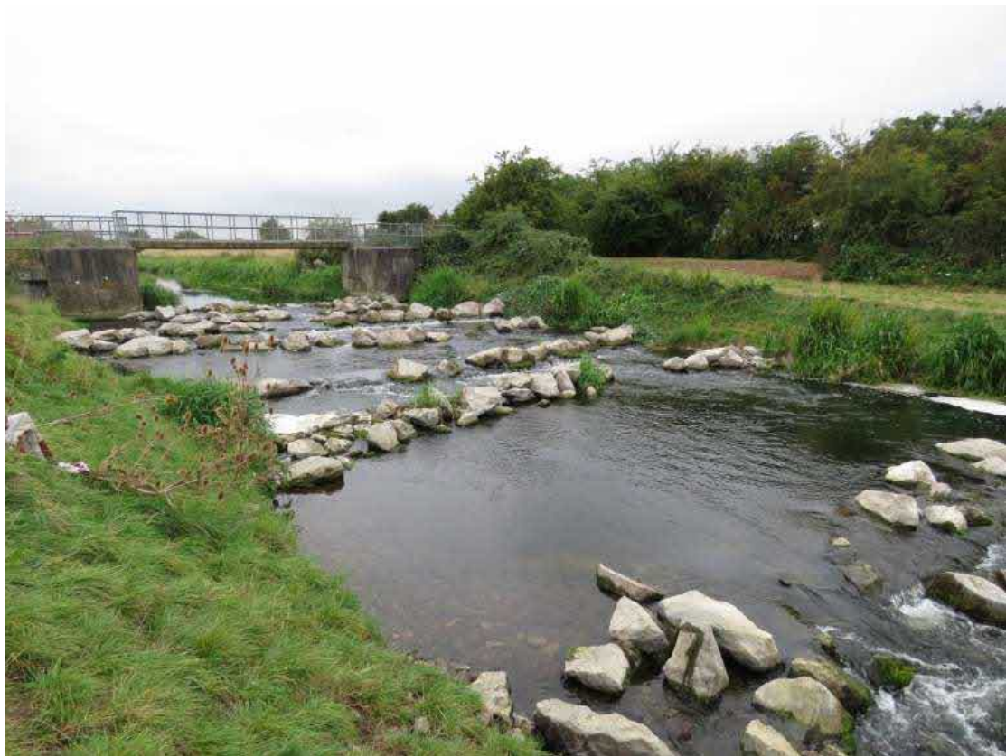
Fig 16. Before (above) and after (below) images of Aubourn Rock Ramp, River Witham, Lincolnshire. A rock ramp fish and eel pass completed nearby to South Ormsby.
