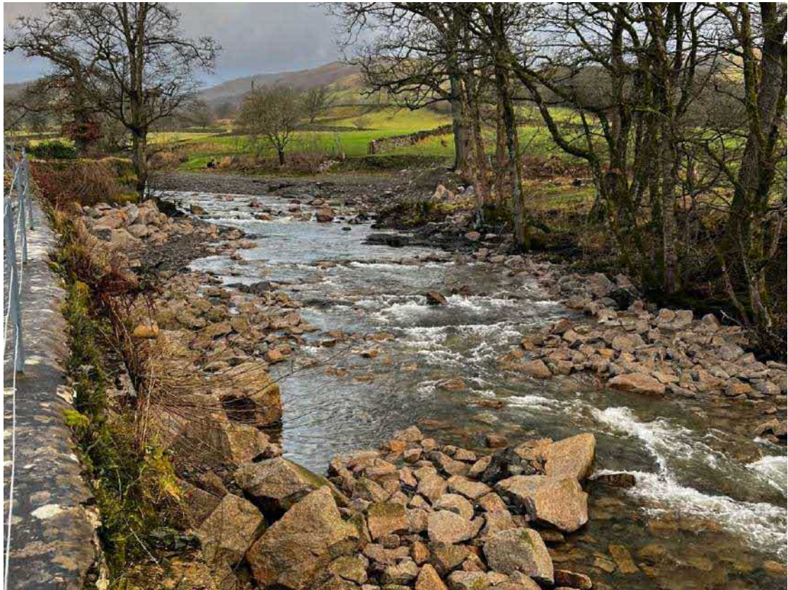
Fig 17. Before (above) and after (below) images of Bowston weir removal, River Kent, Cumbria. A 44% biodiversity net gain was reported following completion of the rock ramp.
