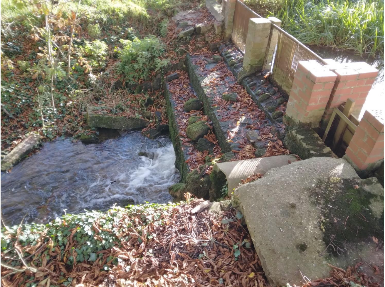
Figure 2 – Current condition of the Weir
