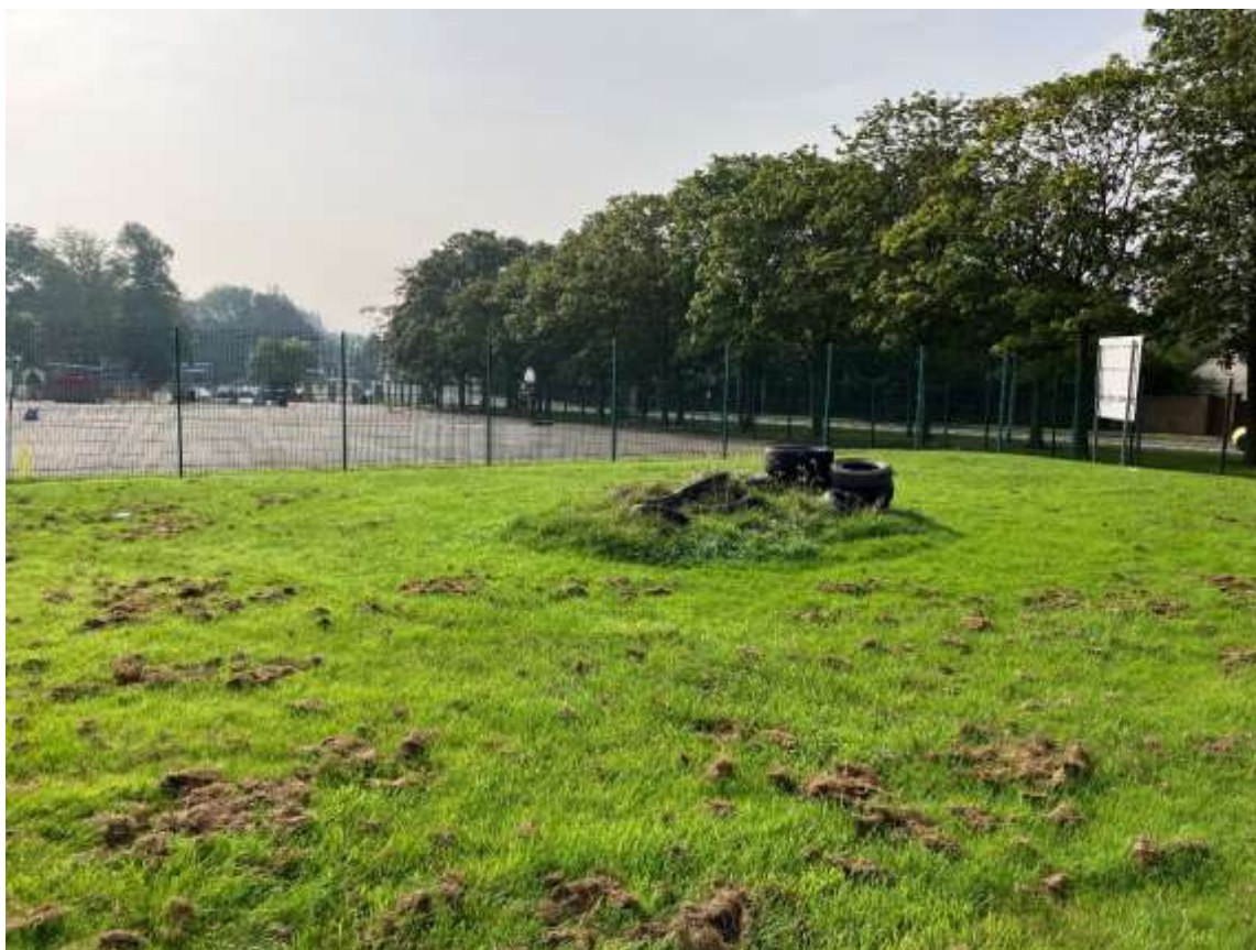
Figure 2-C: Small surface depression with tyres in the southeast of the proposed MUGA area
