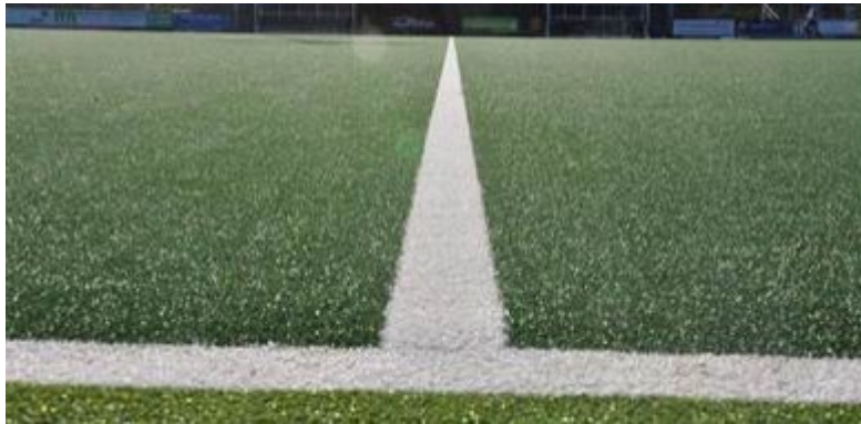
Figure 2 - Typical 20mm 2G Sand-dressed Turf System
