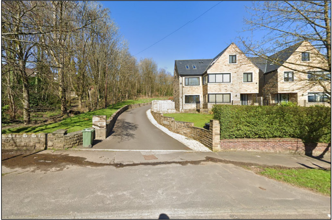
Figure 2.3 – Existing Site Access Arrangements
