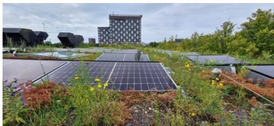
Green roof with inset PVA
