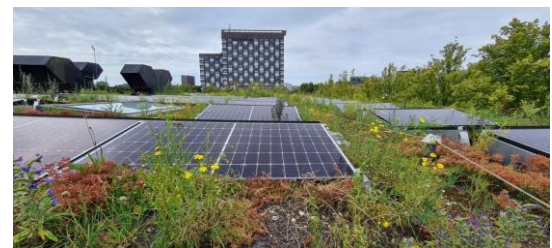
Green roof with inset PVA
