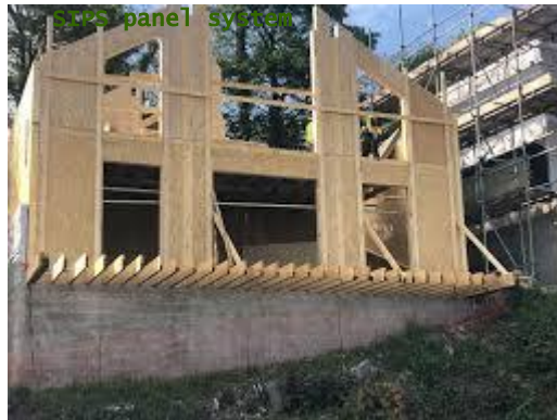
SIPS panel system
