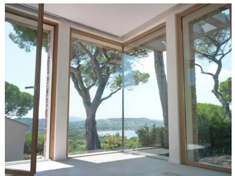
high performance timber windows with integral blinds to manage passive solar gain
